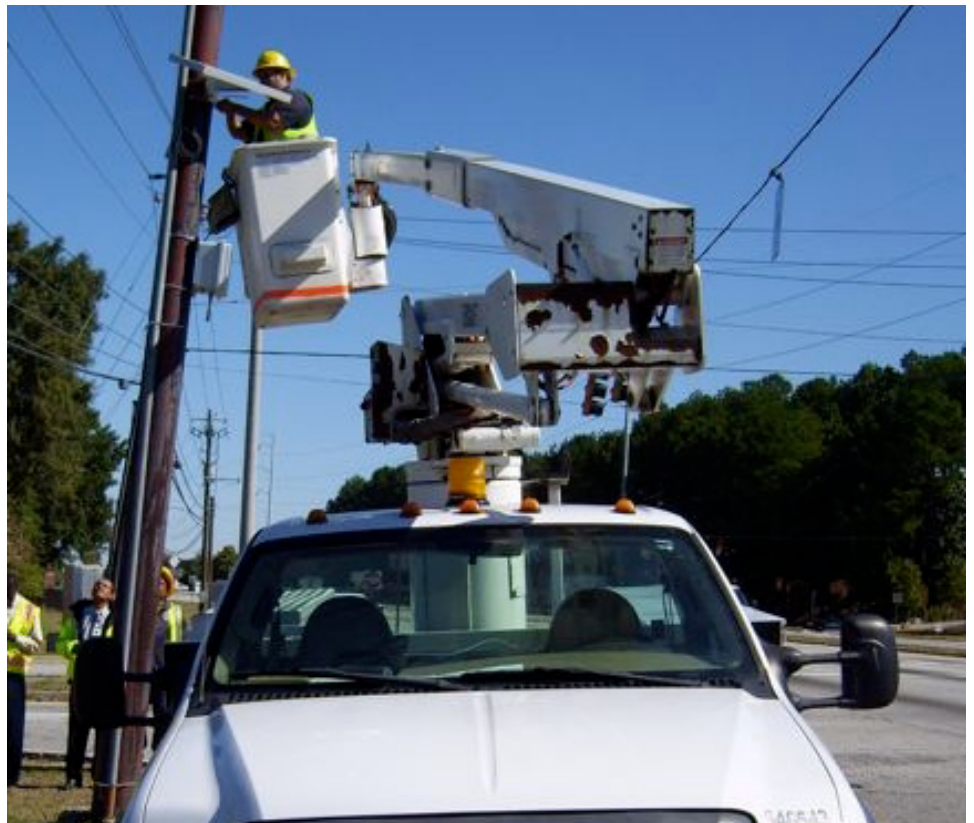
Installation of Solar Self Contained BlueTOAD Unit
